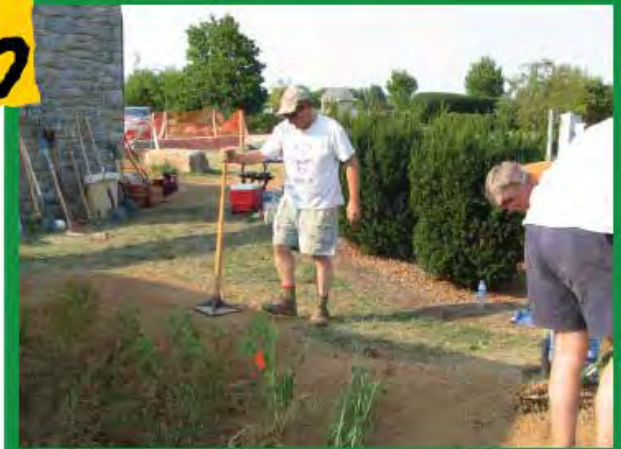
Build & stabilize the berm - include a spillway in the berm! *
